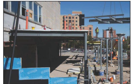
Workers stand by to fasten canopy steel for our new entrance on Bricker Avenue.
