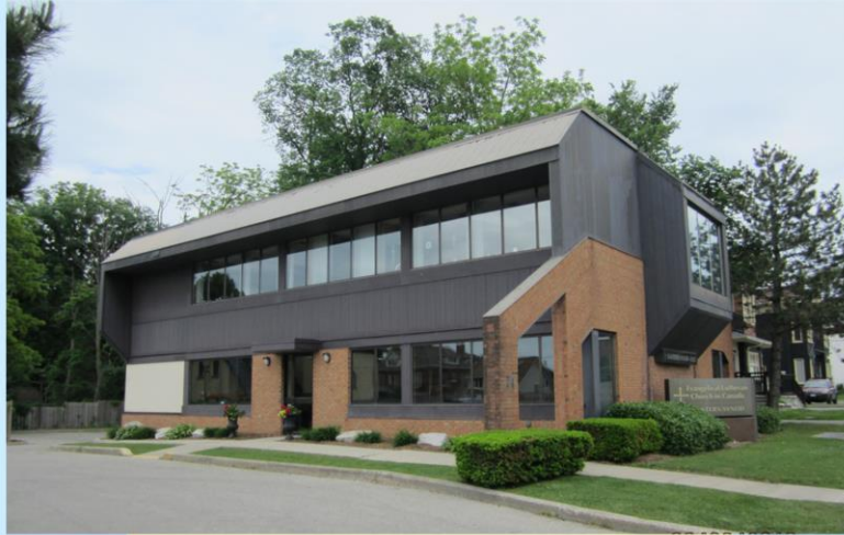
Office, Infrastructure, Supplies
